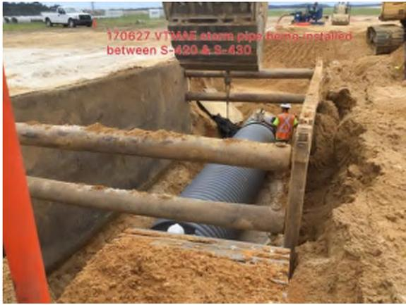
170627 VTMAE storm pipe being installed between S-420 & S-430
