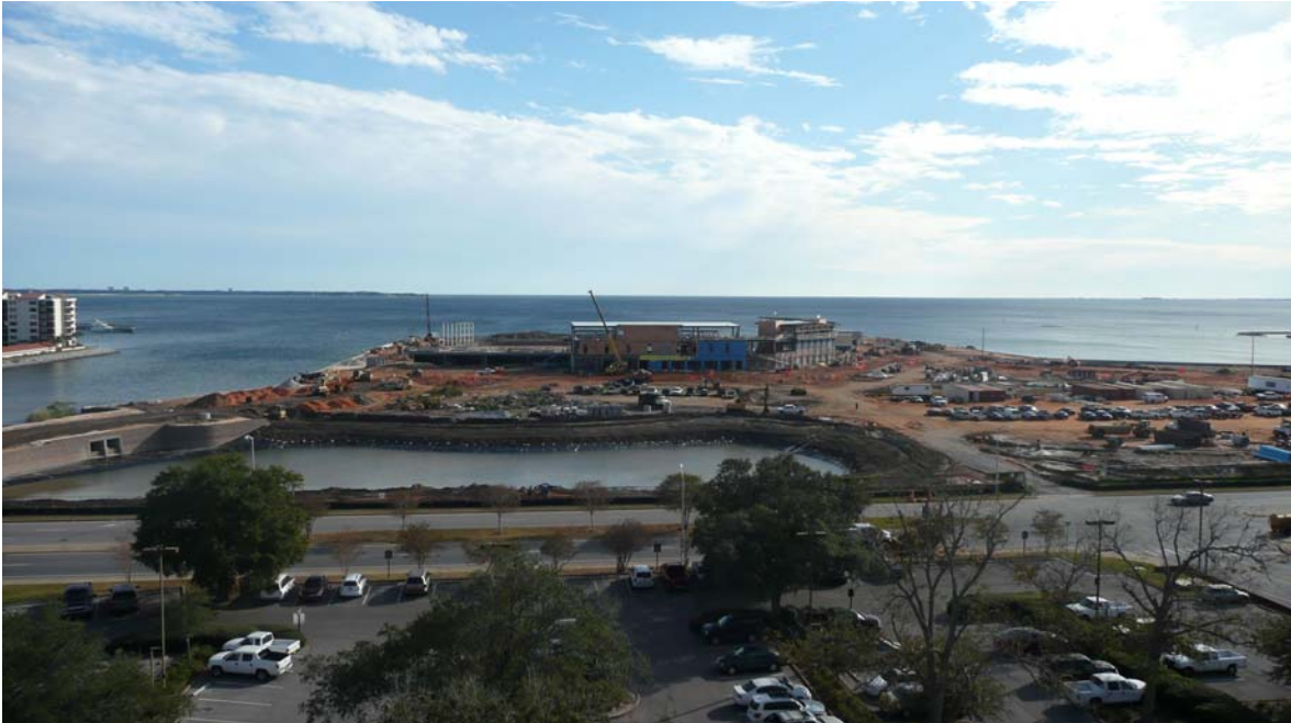
Project Under Construction
